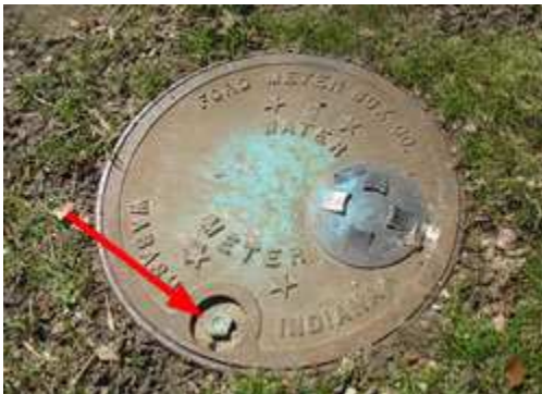
Water meter cover with a pentagon (5-sided) security nut
