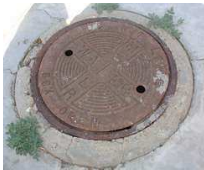
Water meter cover - twist and lift off
