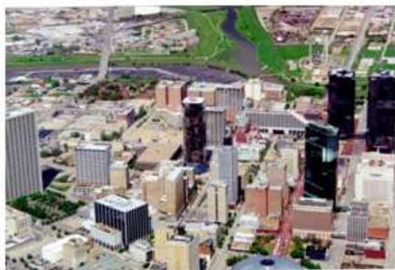
Damage Fort Worth March 2000
