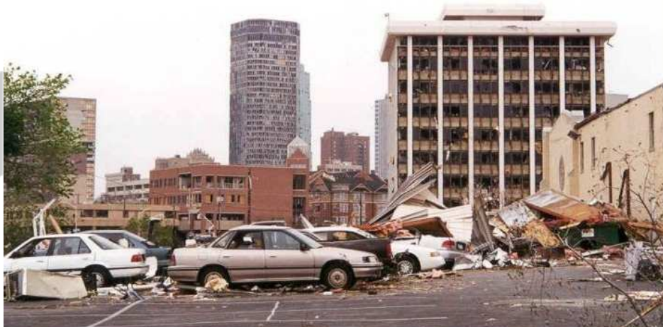
Tornado Damage Fort Worth, TX
