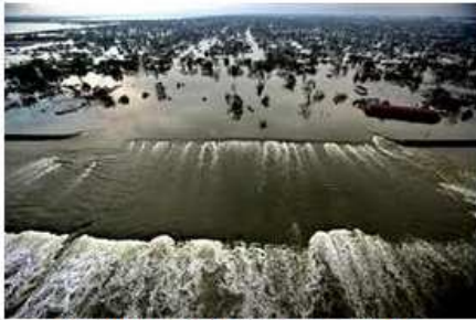
Katrina New Orleans levees topple
