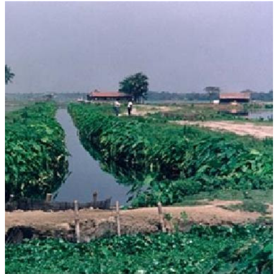
Open channel through which sewage is flown. Lush growth of Colocasia is seen on either side of the channel.
