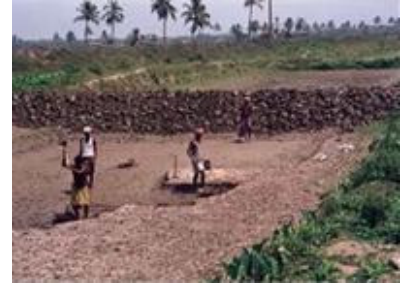
Silt is removed at least once in three years.
