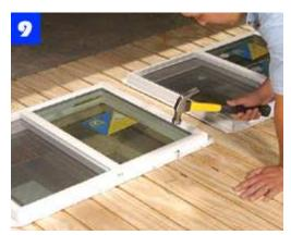
Drop the windows into wall openings and square them with the wall. Fasten them with galvanized roofing nails.
