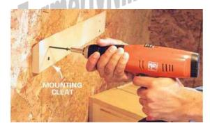
**5.** Position the other half of the mounting cleat about 40 in. Above the work surface and fasten it to the wall studs with four 3-in. screws. Hang the cabinet and drive two 3-in. screws through the bottom 1x 2 into the wall studs for extra strength.
