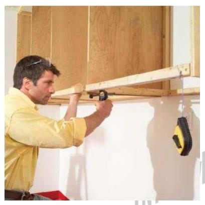
11 String a line along the bottom corner of the front rail. Straighten the rail to the line, clamp it, then screw the panels to the rungs.
