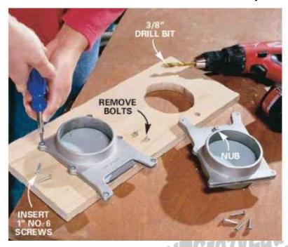
3. Mount the blast gates in the openings. Replace the bolts that hold the two sides of the blast gate together with four 1-in. No. 6 wood screws. Don't overtighten or you'll pinch the gate closed. (Note: We also drilled a 3/8-in. hole to recess a little nub and bolt in the top of our blast gate.)
