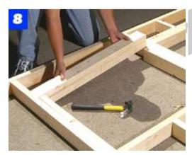
Set the window headers in place on top of the jack studs and secure them by nailing through the king studs.
