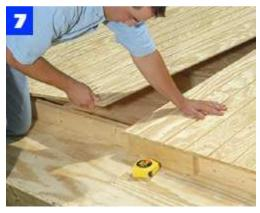
Nail 4 x 8 plywood siding directly onto the studs. Use the siding's factory edges to help square the wall.
