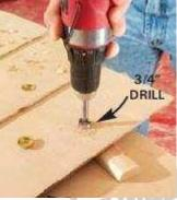
Test-fit all the doors and slide them to the closed position. Mark the best finger pull placement. Then drill 3/4-in. holes and press in the finger pulls. (A dab of polyurethane glue will keep them from popping out.)
