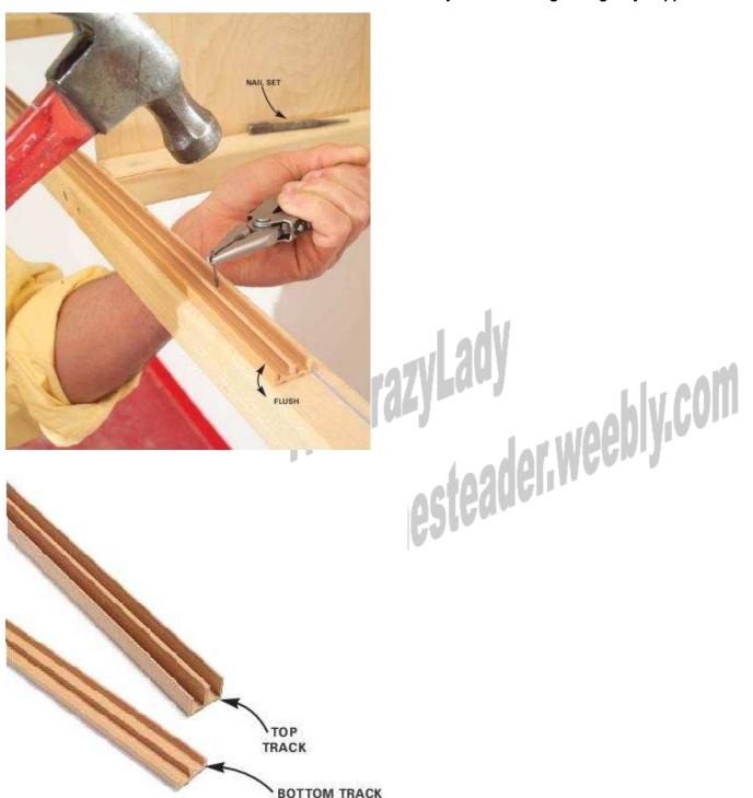
**12** Cut the tracks to length, then tack the bottom track to the bottom rail with 1-in. brads. Punch the brads to the bottom of the grooves with a nail set. Spread polyurethane glue on the top track and tack it into place.
