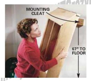
**8.** Level and screw the other half of the mounting cleat to the wall with four 2-1/2 in. screws driven into the wall studs. Hang the cabinet on the interlocking mounting cleats.
