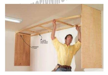
Tack a temporary cleat 1-3/4 in. below the ceiling, rest the top ladder on it, and lift it into place. Screw it to the end panels and then fasten it to any available ceiling framing and to the wall with lag screws.
