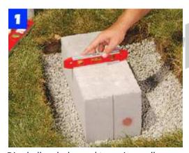
Dig shallow holes and tamp in small-aggregate crushed rock. Level each solid block in both directions.
