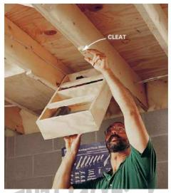
Make the width about 3/8 in. narrower than the cavity it fits in and use double-nutted 3/8 in. x 3-1/2 in. carriage bolts for the two pivot points. Two plywood cleats pivot on 3-in. screws to hold each drawer in place in the "tucked" position. The drawers are perfect for anything you only need occasionally. But be careful to keep contents relatively light so you can safely open and close the drawers. It's definitely not the place to store your anvils.
