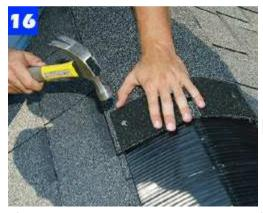
After nailing the ridge vent over the gap left at the peak, install cap shingles by nailing through the spacer tabs.
