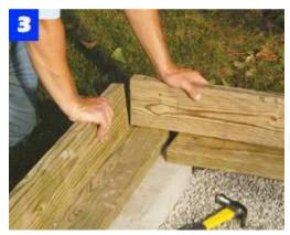
Build the sill box with treated 2 x 6 lumber. Stagger the sills and band joists so they overlap at the corners.
