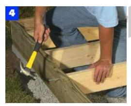
Set the floor joists in place, crown edge up, and nail them through the band joist with 16d galvanized nails.
