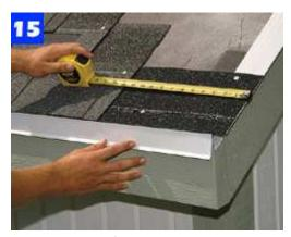
Prepare the roof with drip caps and a starter strip. Offset each row of shingles and run the edges 1/4 in. long.
