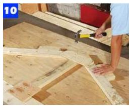
Make a truss jig on a piece of plywood. Glue and nail the corners together with 1/2-in.-thick plywood gussets.
