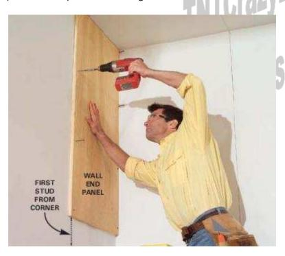
**2** Press one end panel against the ceiling and the rear wall and screw it to the corner and first wall stud. Angle the back screws slightly to catch the corner stud.
