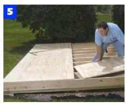
Deck the joists with 3/4-in. tongue-and-groove plywood. Stagger each sheet and secure with 8d nails.
