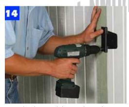
Hang the door with heavy-duty T-hinges, using longer screws in the doorjamb. Then, install a lockable latch.
