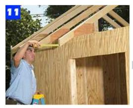
Install the end trusses, then stretch a string between them. Use the line to help position the remaining trusses.
