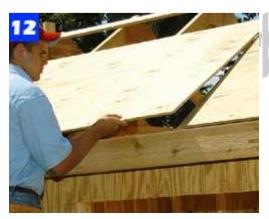
After adding the blocking and fascia at the gable ends, cover the roof with 1/2-in. plywood. Secure it with 8d nails.
