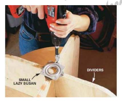
**6.** Screw the bottom ring of the 3-in. lazy Susan to the dividers on top of the bin with 3/4-in. screws. Assemble the support shelf. Mark the bin rotation center on its bottom (about 13 in. from each wall) so the bin will clear the wall by about an inch when it rotates.
