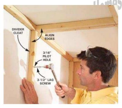
Nail the divider wall cleats to the studs, then predrill three evenly spaced 3/16-in. pilot holes and bolt the cleats to the studs with 3-1/2 in. lag screws.
