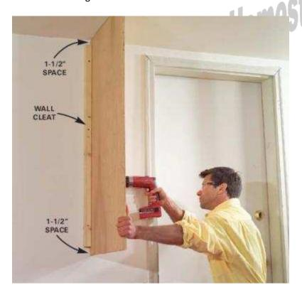
4 Press the end panel against the ceiling and wall, then screw it to the outside edge of the wall cleat with 2-in. screws.
