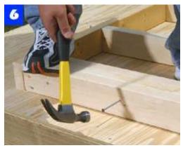
Nail three studs together at both ends of the long walls. You'll nail the end studs for the short walls to these.
