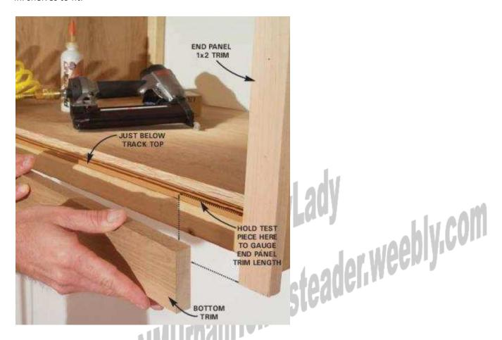
17 Cut 1x2 end panel trim to extend about 3/4 in. below the end panel. Nail into place. Cut and nail 1x3 trim for the top and bottom rails.
