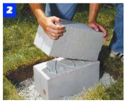
When stacking solid blocks to accommodate a sloping grade, glue them together with construction adhesive.
