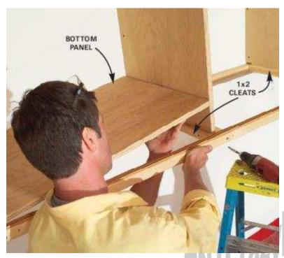
13 Cut 1x2 cleats and screw them to the bottom of the divider panels to support the bottom panels. Cut the bottom panels to butt against the door track. Screw them into place.
