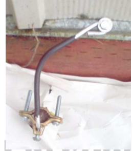
A common steel garden shed, grounded using 1/4" ground wire: The insulated ground wire does not touch the base/floor of the shed so things inside are safe.
